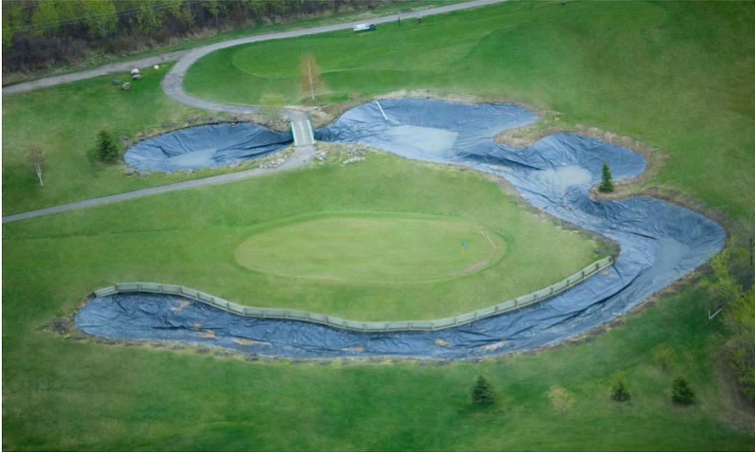
A common construction technique to provide either primary or secondary containment is the construction of a lined earthen pit. It is more complex than simply digging a hole in the ground as several factors need to be considered during the design process.
